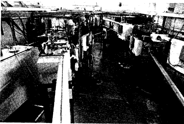
Fig. 3 View of present transfer hall installation.
