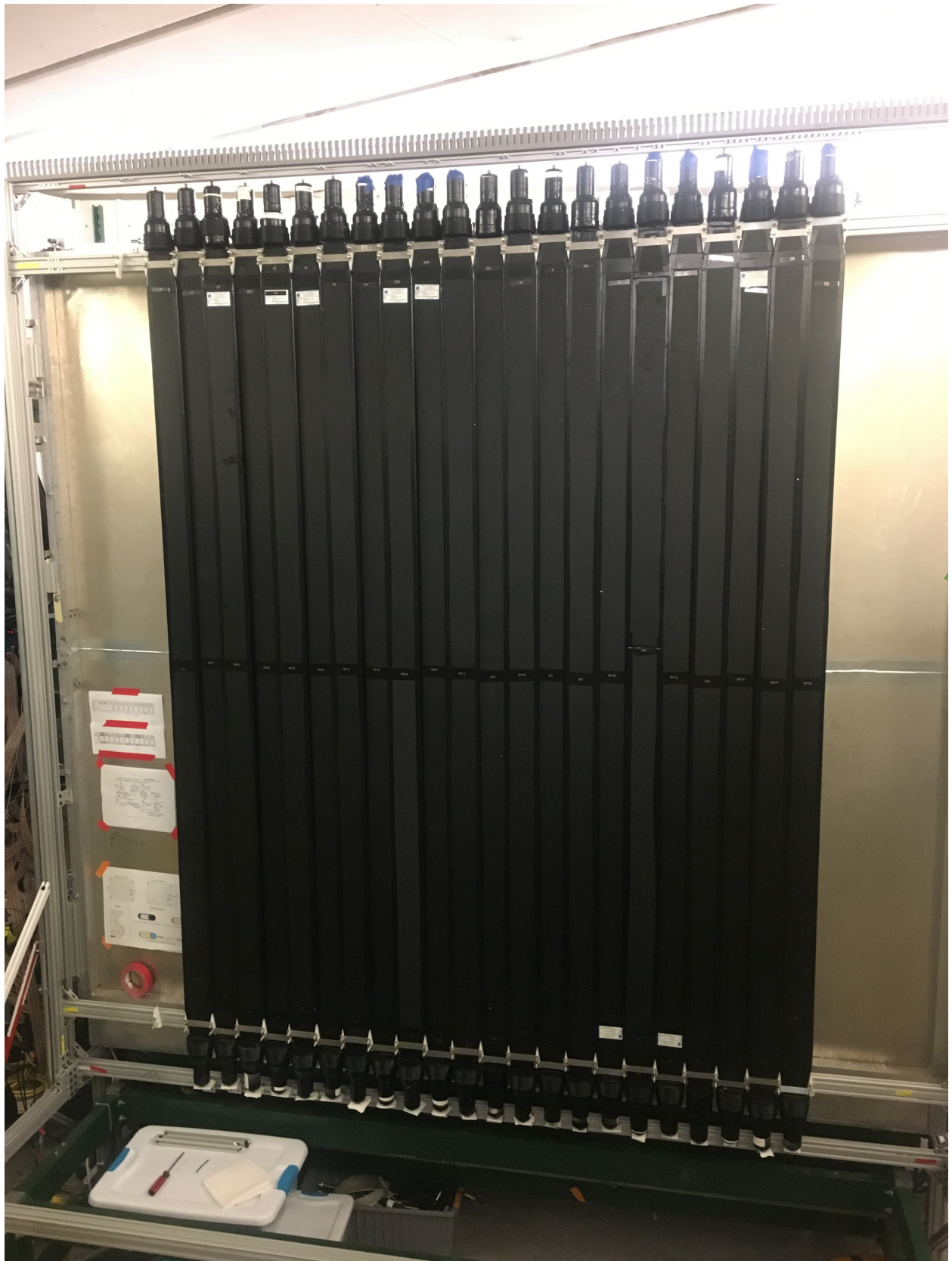
Figure 2.22: Charged-particle Veto Wall construction in progress. 22 bars have been installed in place.
