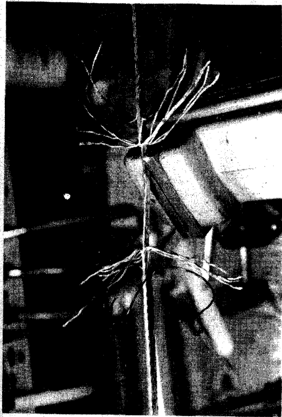
Fig. 3. Conductor splice in process.
