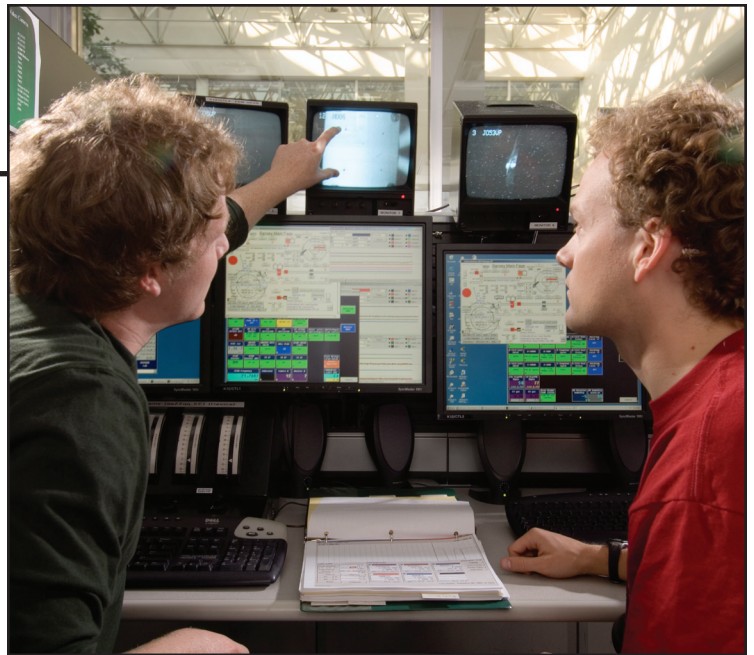
Operators use video monitors and computer terminals in the control room to monitor and operate the cyclotrons and beam lines.
