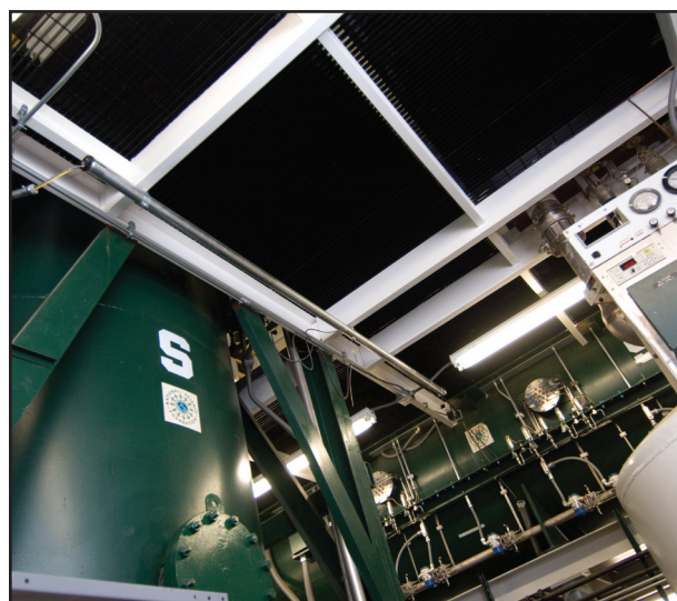
Two views of the main distribution box. This is the center point for sending cryogenics to the rest of the lab.
