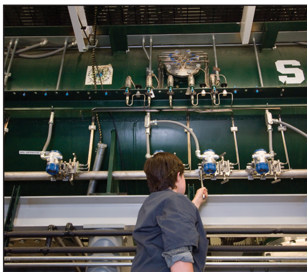
Two views of the main distribution box. This is the center point for sending cryogenics to the rest of the lab.
